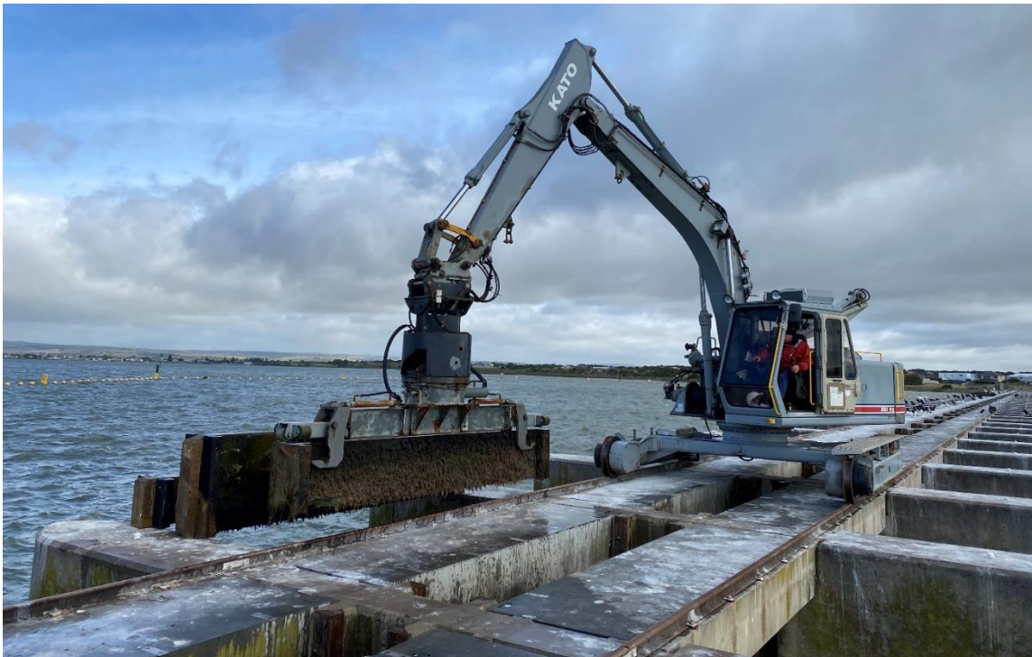
Figure 2: A stop log being pulled from the Goolwa barrage as part of an audit being undertaken by SA Water (Qifeng Ye, SARDI)
